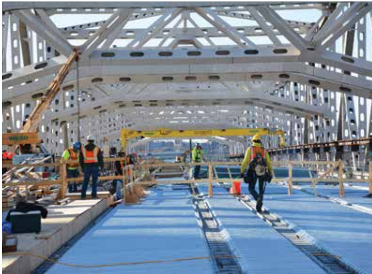
Nearly 700 crew members have worked on the Downtown Crossing project since construction began. As part of the renovation, more than 3.5 million pounds of old steel are being removed from the Kennedy Bridge, with new steel being installed.
