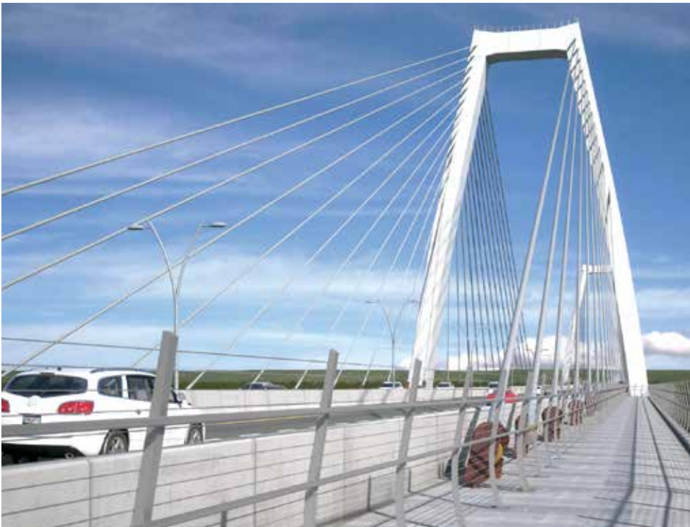
The East End Crossing features a new bridge spanning 2,500 feet across the Ohio River. The two main towers are 300 feet tall with 104 stay cables supporting the bridge deck.
